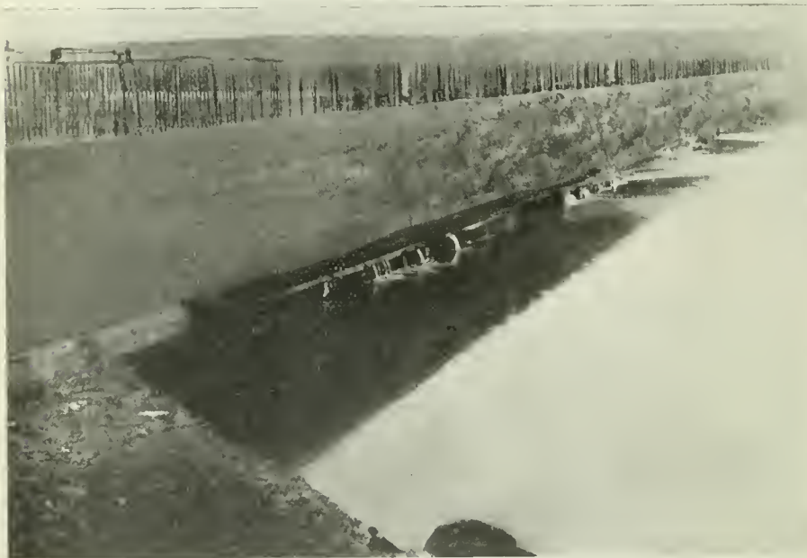
Fig. 2.—West side of cement pond showing leakage of water. Over the ironrods at the upper left hand corner of the illustration can be seen the gearing of the rearing apparatus inside of the cement pond.
